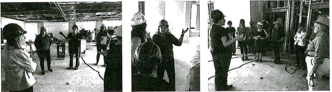
CIMCO held its April meeting in Galesburg and the highlight of the meeting was a tour of the new Galesburg Public Library, which is currently under construction.
